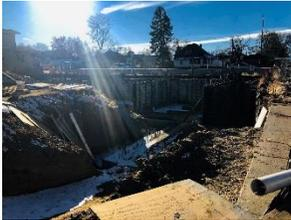
The Hilltop development project (located on Broadway at Lehigh Ave.) is currently progressing through the foundation construction. The footings for the foundation have been poured; the walls are being framed and should be constructed by the second week in December. Upon completion of the wall construction, the public sidewalk will be reconstructed and opened to the public.
