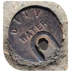
**How do I extend the stop box to grade?** The vertical access pipe on the curb stop valve in front of your home comes in two parts: a larger diameter pipe and a smaller diameter pipe. They are threaded together so the top part can be moved up and down. To adjust the valve box so the lid is even with the surface of the ground, dig down until you can rotate the box up or down as needed.
